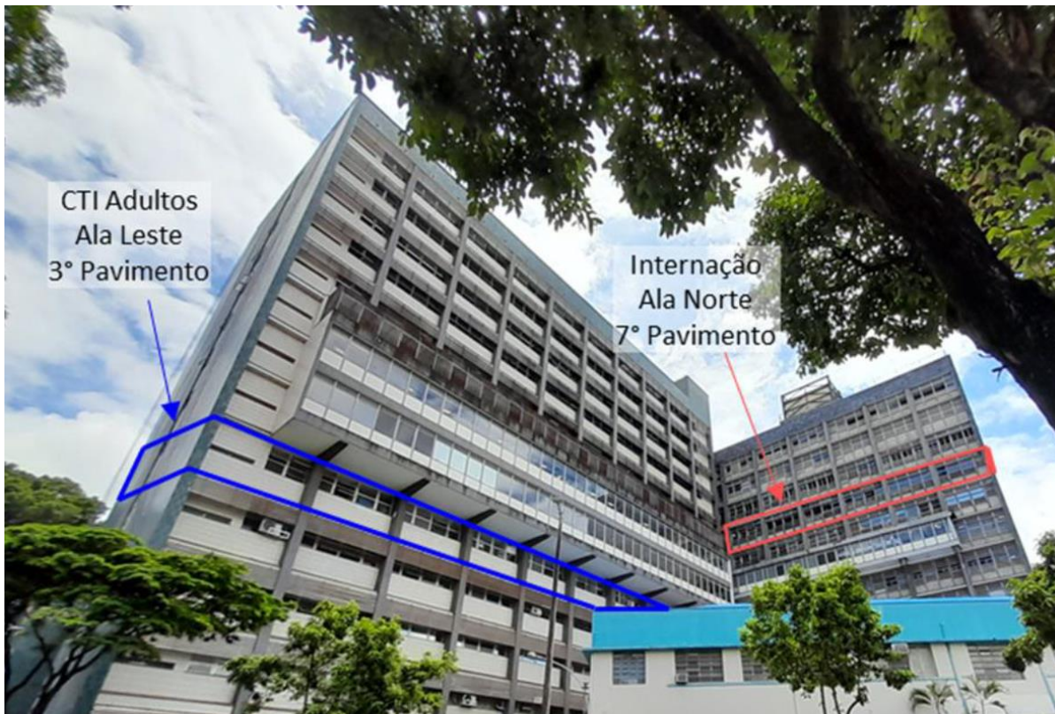
Figure 1: Identification of the hospital wings analyzed in the case study.
